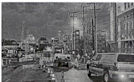
WATER ASSET MANAGEMENT
