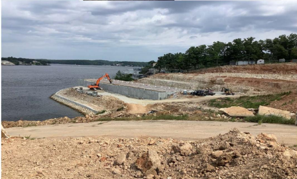
Topsider Condos under construction
