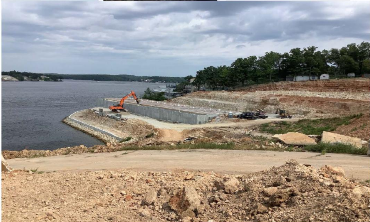
Topsider Condos under construction
